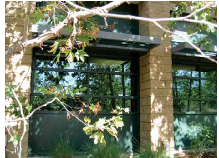
Lower-floor windows are thought to be more dangerous to birds because they are more likely to reflect vegetation. Photo by Christine Sheppard, ABC
