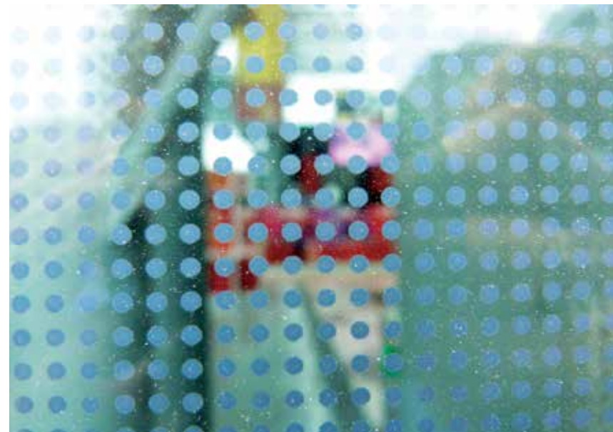
At close range, a visible pattern of frit dots breaks up reflections, making the glass safe for birds. Photos by Glenn Phillips, ABC
