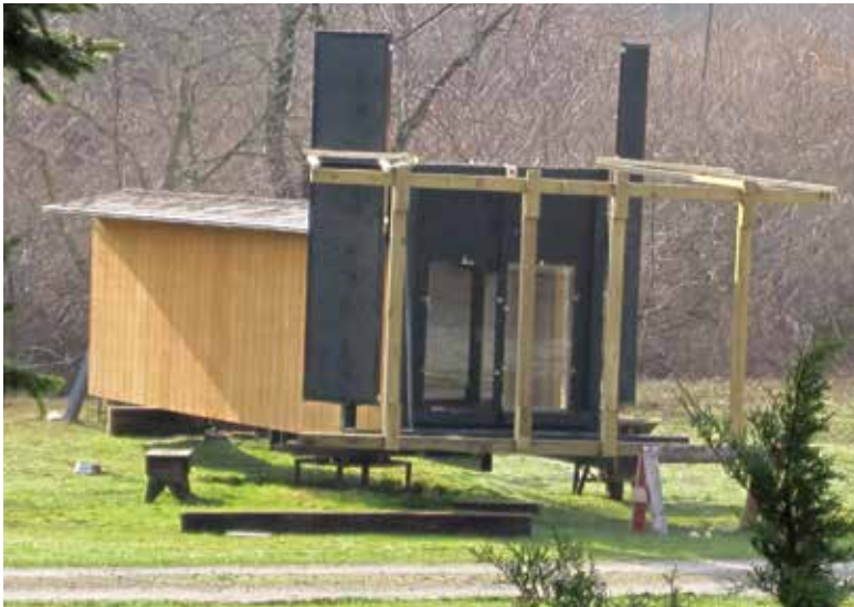
The tunnel at Powdermill, showing the framework where the background will be mounted. Photo by Christine Sheppard, ABC
