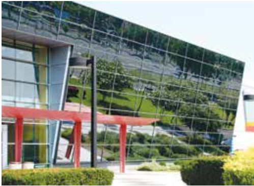
Reflections in this angled façade can be seen clearly over a long distance, and birds can approach the glass from any angle. Photo by Christine Sheppard, ABC
