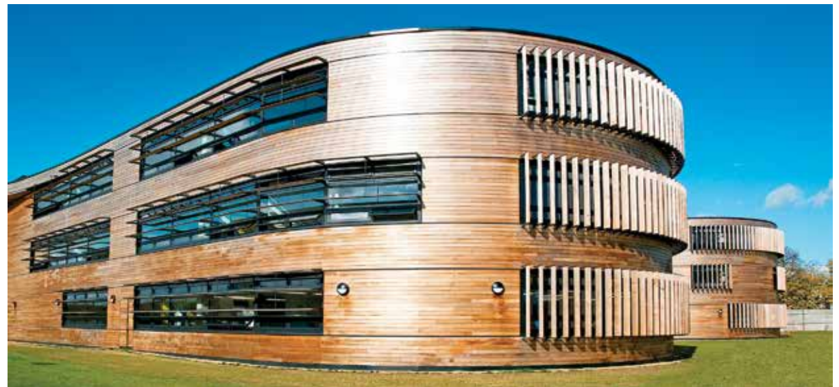
For the Langley Academy in Berkshire, U.K., Foster + Partners used louvers to control light and ventilation, also making the building safe for birds. Photo by Chris Phippen Ofis
