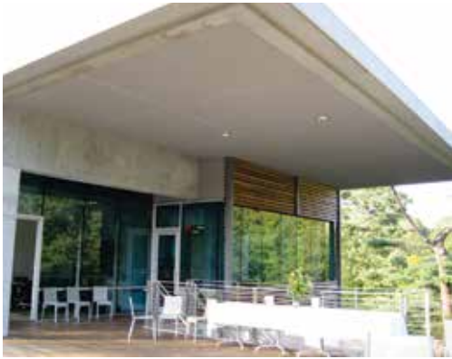
Overhangs block viewing of glass from some angles, but do not necessarily eliminate reflections. Photo by Christine Sheppard, ABC
