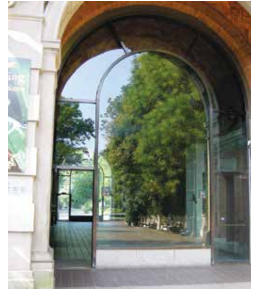
Large facing panes of glass can appear to be a clear pathway. Photo by Christine Sheppard, ABC
